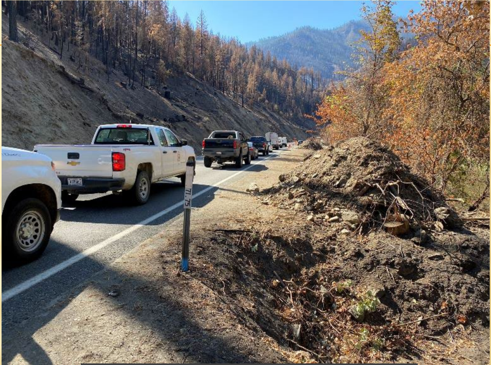
Erosive slopes along highway 96 in the HEAD fire
